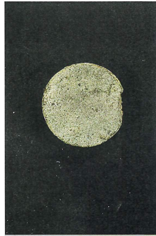
TH #4 Top of Asphalt Pavement Ø = 150 mm
