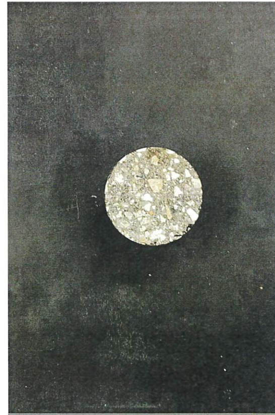
PC #4 Top of Asphalt Pavement Ø = 100 mm
