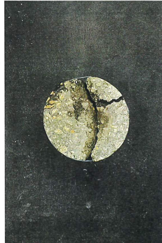
Th #12 Top of Asphalt Pavement Ø = 150 mm
