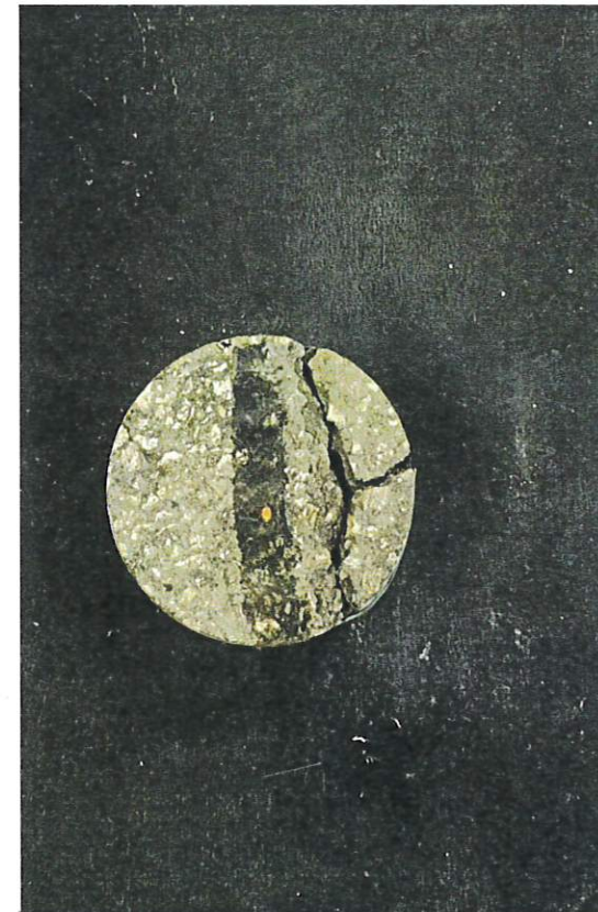
TH #9 Top of Asphalt Pavement Ø = 150 mm
