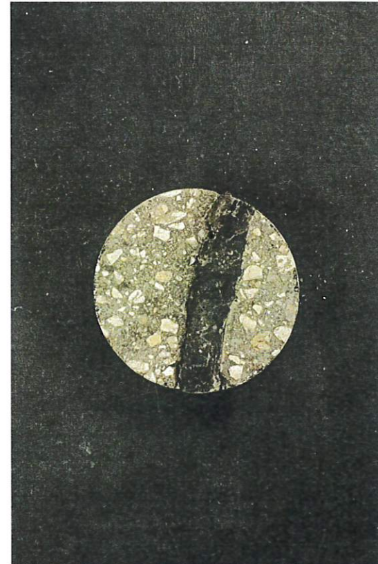
PC #21 Top of Asphalt Pavement Ø = 150 mm
